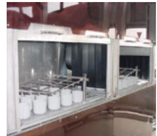
Waste Reagent Treatment Facility
