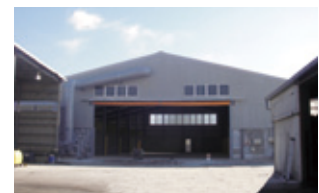
Fermented Compost Facility
