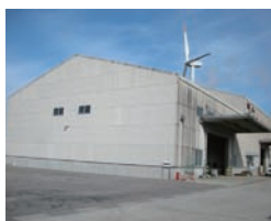
Kitakyushu Hibiki Plant
