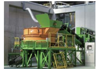
Manufacturing Facility for Cement Raw Material
