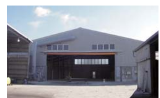
Fermented Compost Facility
