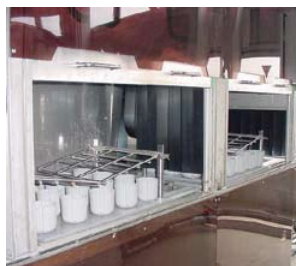
Waste Reagent Treatment Facility
