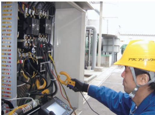
We use electricity monitors to perform surveys and analyses of the current status of power used, and promote the optimization of operating conditions.
